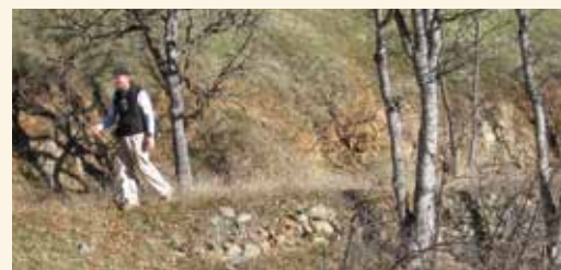
Impressive stonework is found in retaining walls which still support the trail in many places along the ditch.
